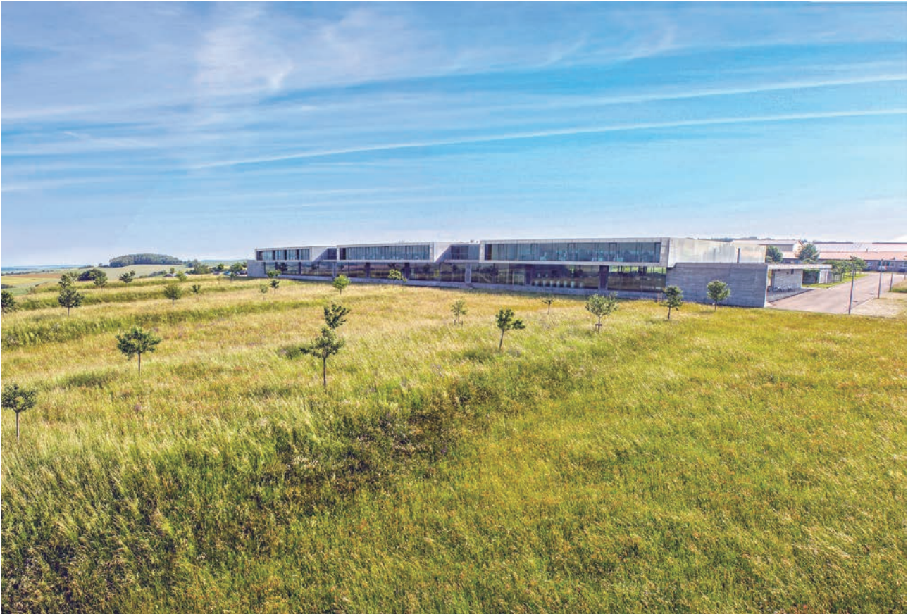
BASS GmbH & Co. KG's headquarters in Niederstetten, Germany. Since its founding in 1947, BASS has focused on the development, production and sales of powerful threading tools. In 2019, BASS was acquired by OSG Corporation to reinforce its strength in the European market, global affiliated companies and OEMs.
